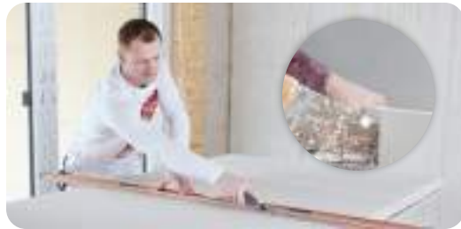
From onsite manual cutting of boards...
